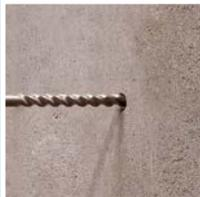
**1** Pre-drill a pilot hole completely through using an 8mm masonry drill bit.
