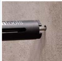
**2** Attach the Deep Cut Core Bit and place the centring guide into the pre-drilled hole. Begin cutting.
